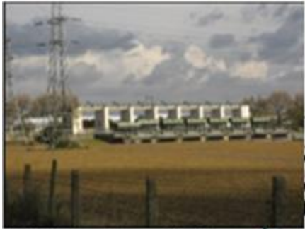
Tail Sluice - One of the biggest pieces of flood risk infrastructure in the country. Part of Ely Ouse Flood Protections Scheme. Allows discharge from Relief Channel at low tide.
