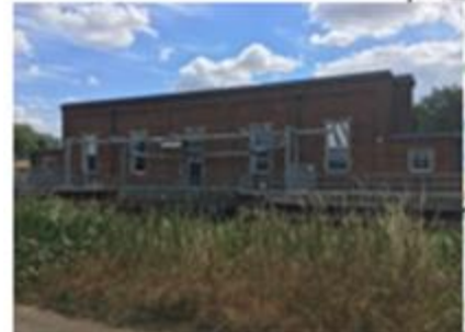
Welches Dam Pumping Station – pumps water from the Counter Drain when gravity discharge not possible.
