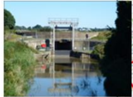
Old Bedford Sluice – water from Counter Drain can discharge at low tide.
